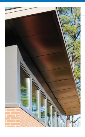
A strong collaboration of simple elegance and modern practicality define our soffit panels and plate wall system. Featuring a clean-line aesthetic, the structure is installed using a unique track and compression channel that allows the panels to be installed in virtually any order. Panels can be removed individually, allowing for easy future access or replacement. Joints are caulked.
